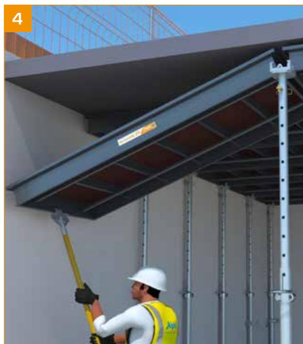
4 - Remover o painel com a sonda HorizontalAL.
