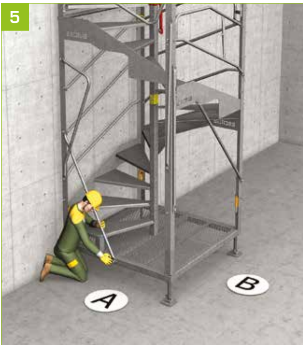
- At the entrances, position the rails, prioritising the main entrance on side A [the sides are indicated on the self-adhesive label].
