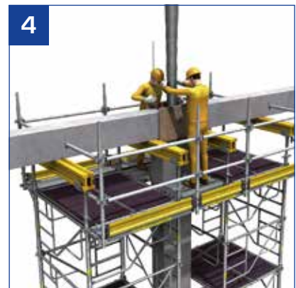
- The decking is assembled with collective safety from a floor level in a temporary position.
