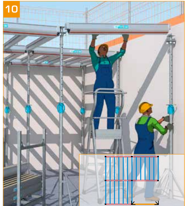
- Set up another primary beam on ST.
