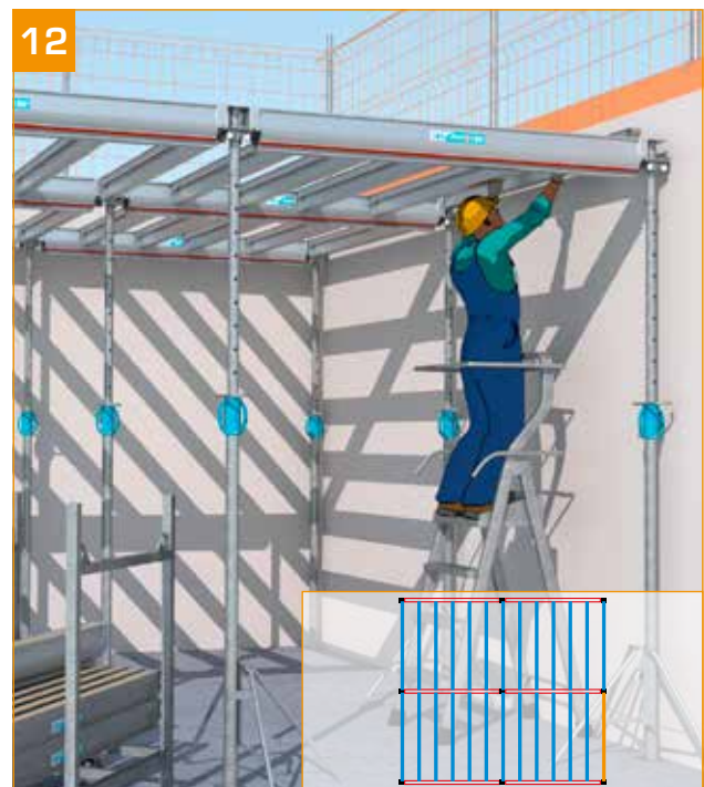
- Finish setting up the secondary beams.
