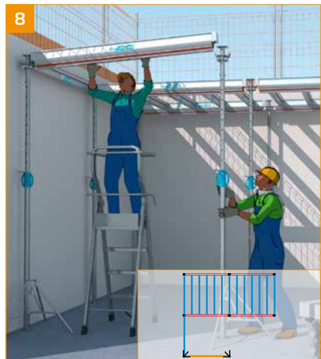
- Set up another primary beam on ST.
