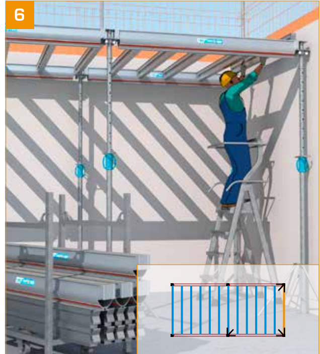
- Finish setting up the secondary beams.
