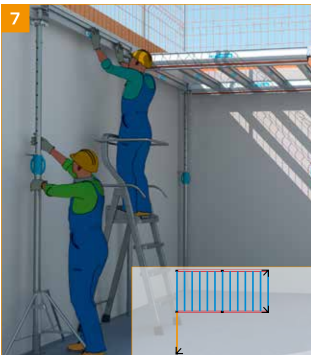
- Set up another secondary beam on ST.
