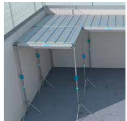
The extendable beams let you go near the cell edges
