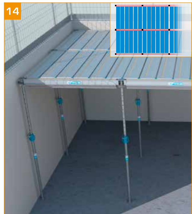
- Continue to mount Eco+ panels+ progressively using the TopPerche Eco, from one to the next.
