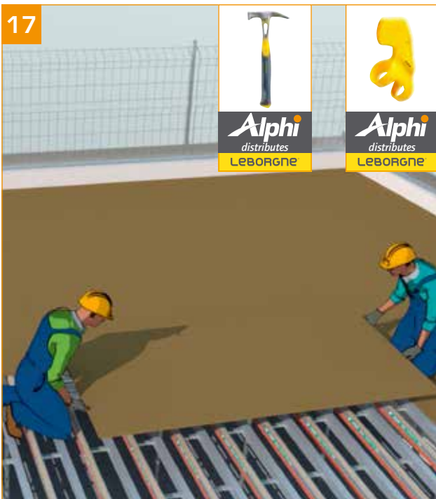
- When the structure is finished and the height has been adjusted: lay the plywood. - Use the plywood cutting support (see Accessories p. 9-10). → Peripheral safety (skin, girder, etc.) ensured beforehand. → Use of the plywood cutting support.
