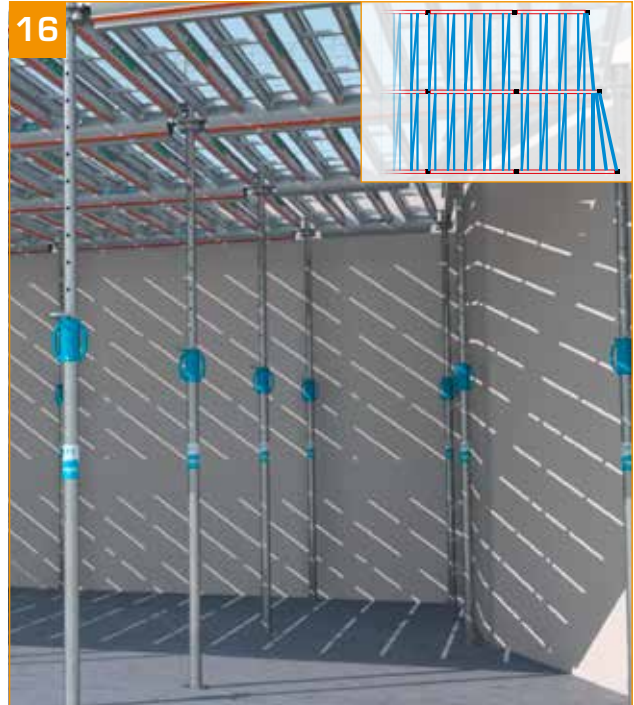
- Adjust the level using a laser level, ST by ST. - A gauge stick hanging from the formwork allows laser adjustment to be performed by one person. - Conduct a final head locking check at this stage.
